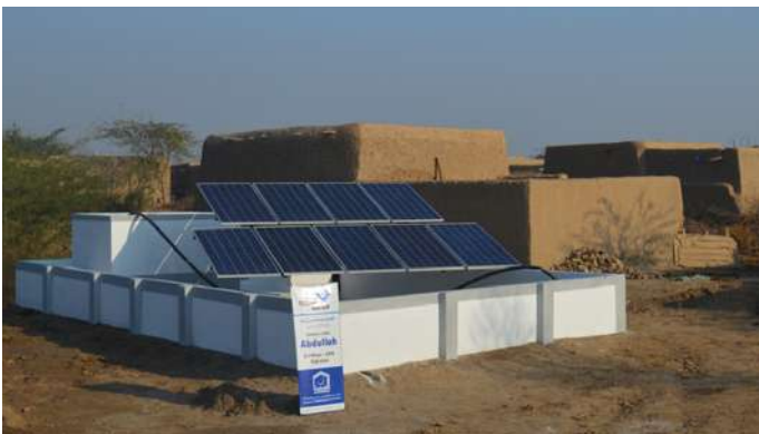
A view of solar water tank project in D.I Khan
