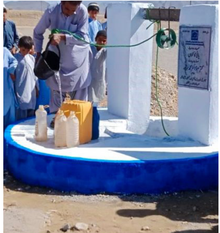
A view of Water Well in Balochistan
