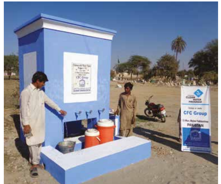
Submersible Water Pump in Khyber Pakhtunkhwa
