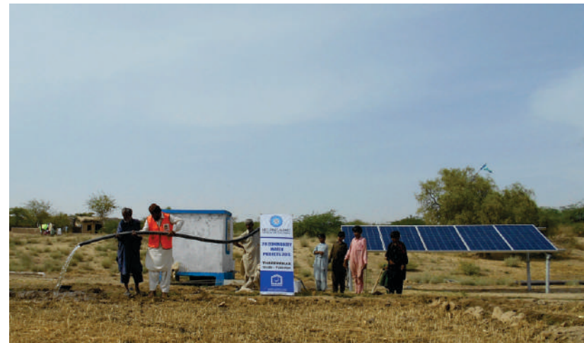
Solar water filtration plant of Alkhidmat Foundation in Tharparkar
