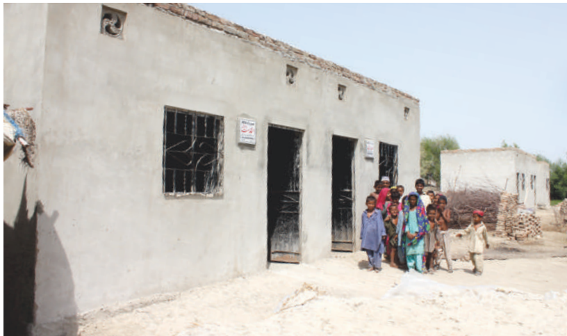
Single room houses for the flood affected people in Sindh
