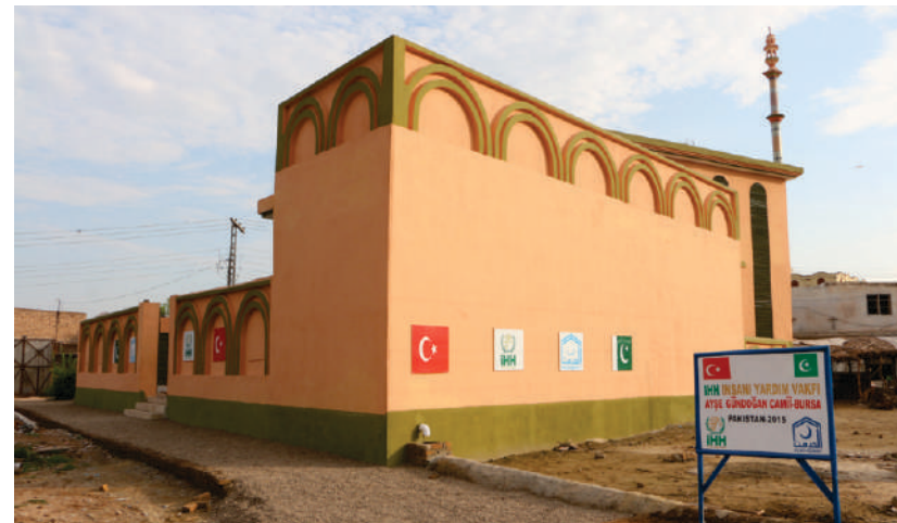
A newly constructed Masjid at Peshawar
