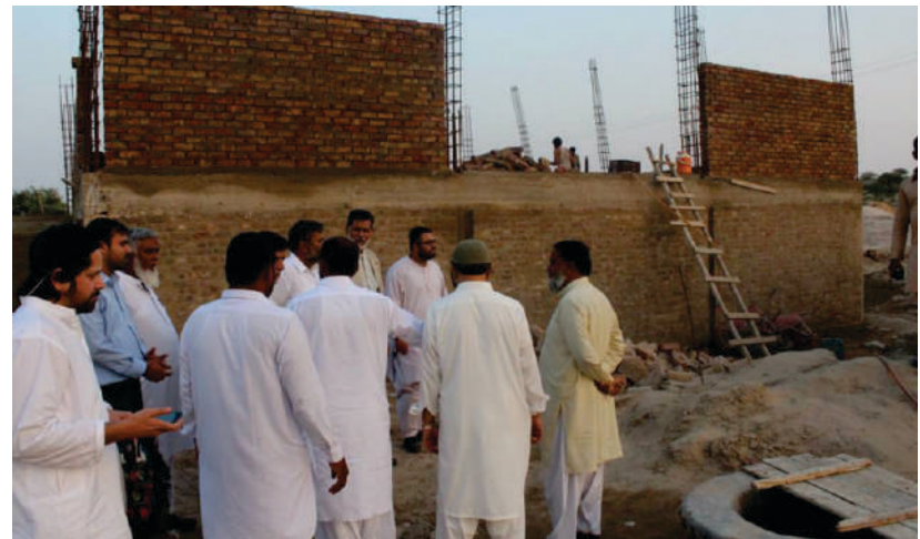
Under construction building of Alkhidmat Thar complex
