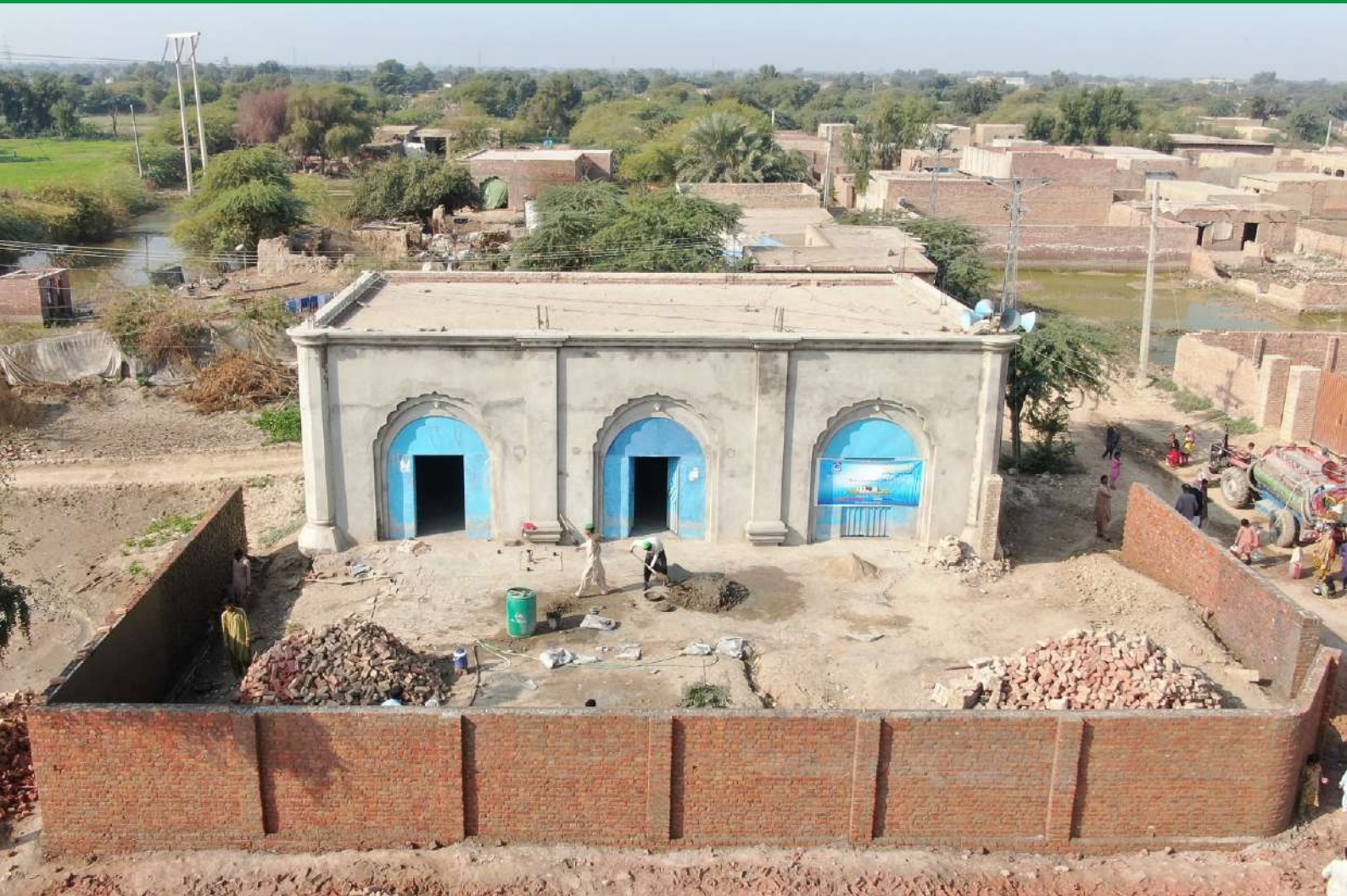
Flood-damaged Masjid being rehabilitated in South Punjab.
