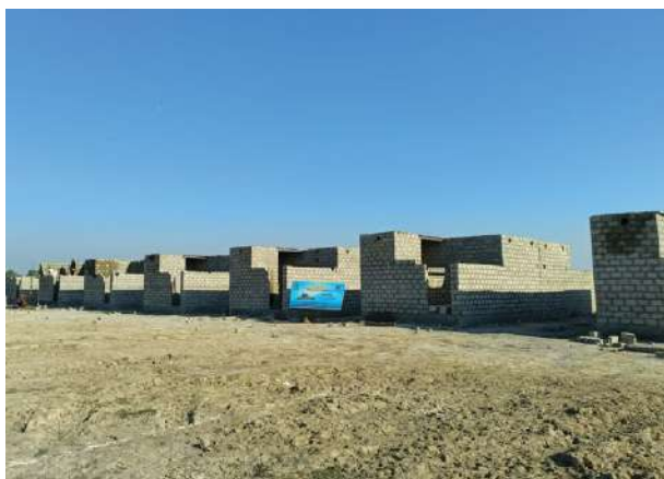
A 40-house model village under construction in Naseerabad, Balochistan.
