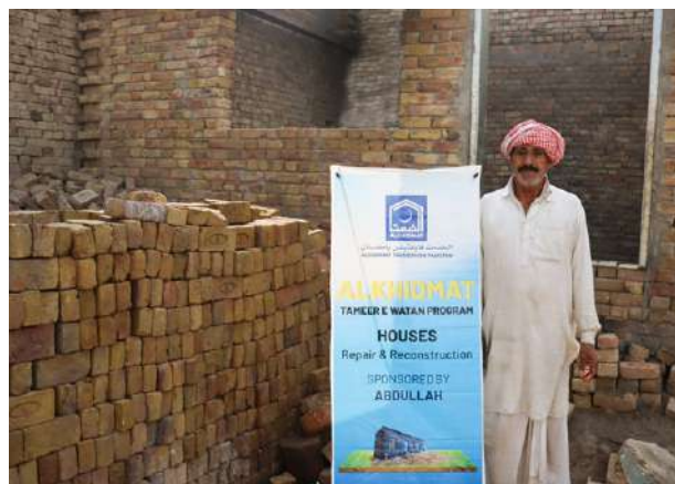
Flood-damaged house being reconstructed in Sindh.
