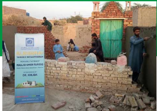
Flood-damaged Masjid is under reconstruction in Naseerabad, Balochistan.
