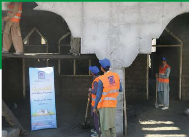
Flood-damaged Masjid is under reconstruction in Gilgit Baltistan.
