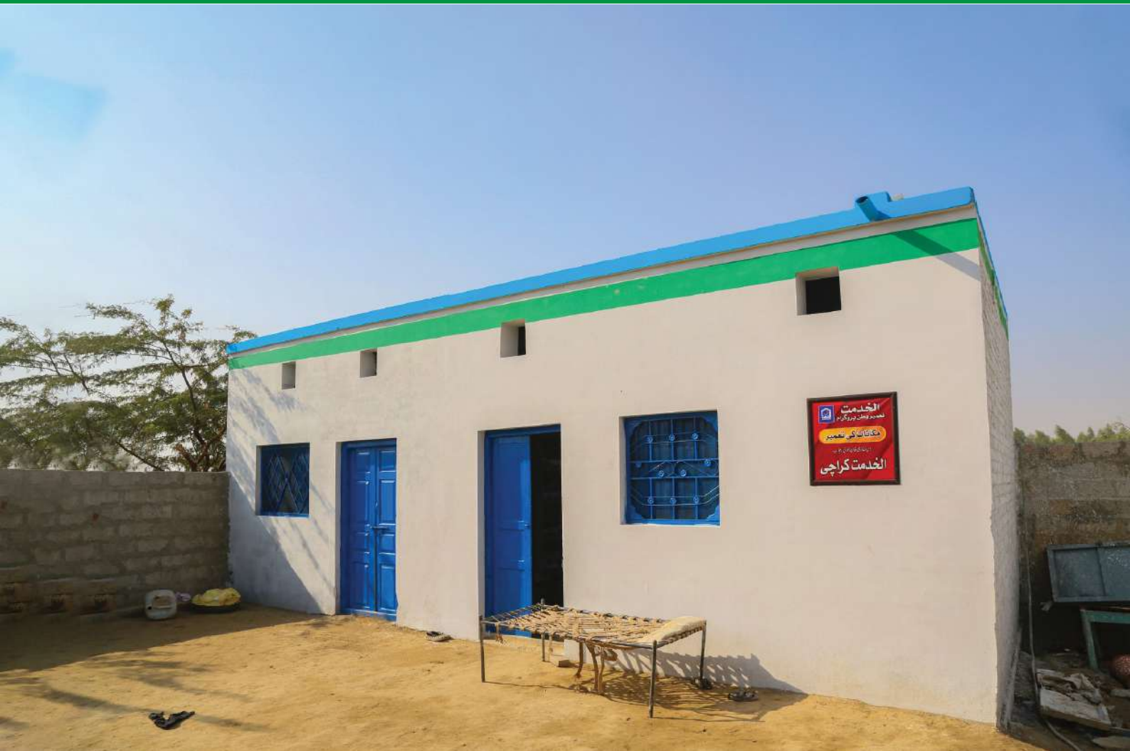
Flood-damaged house reconstructed in Dera Ghazi Khan, South Punjab.
