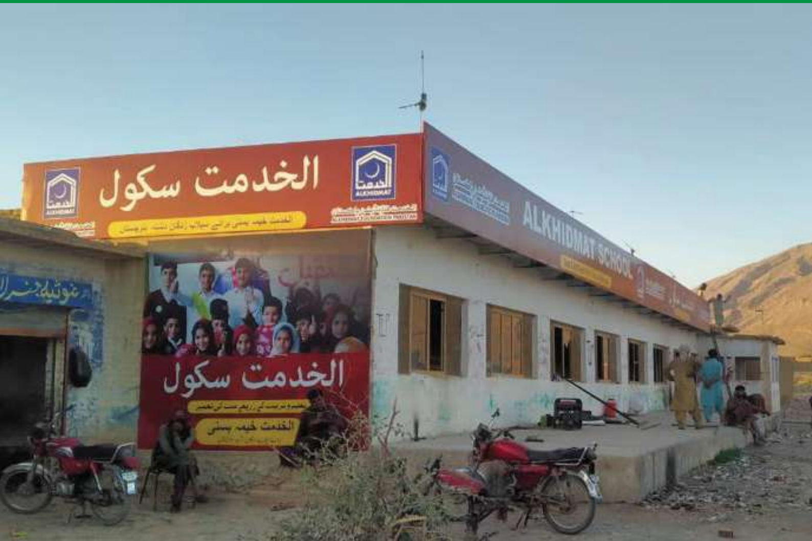
Flood-damaged school rehabilitated in Balochistan.
