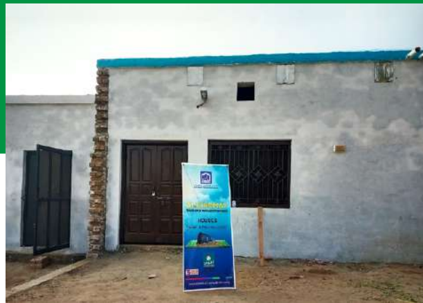
Flood-damaged house being reconstructed Dera Ghazi Khan.
