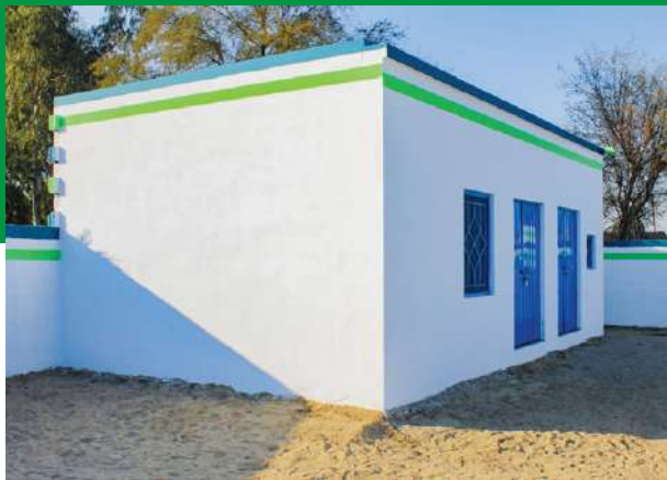
Flood-damaged house reconstructed in Dera Ghazi Khan.
