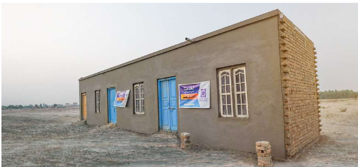
Flood-damaged house reconstructed in Sindh.
