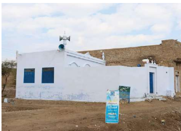
Masjid has been completed in Fazalpur, South Punjab.
