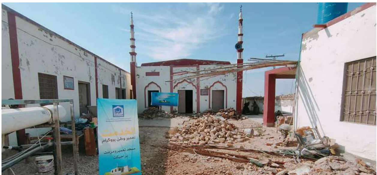
Flood-damaged Masjid is under reconstruction in Balochistan.
