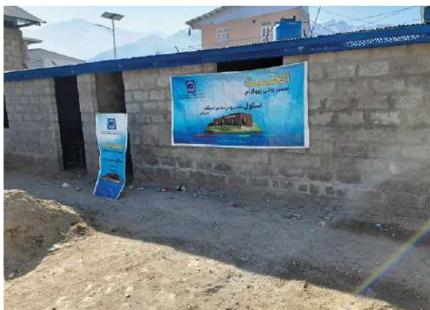
Flood-damaged school is under reconstruction in Dir Upper, KP.
