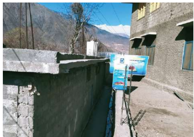
Flood-damaged school is under reconstruction in Chitral, KP.
