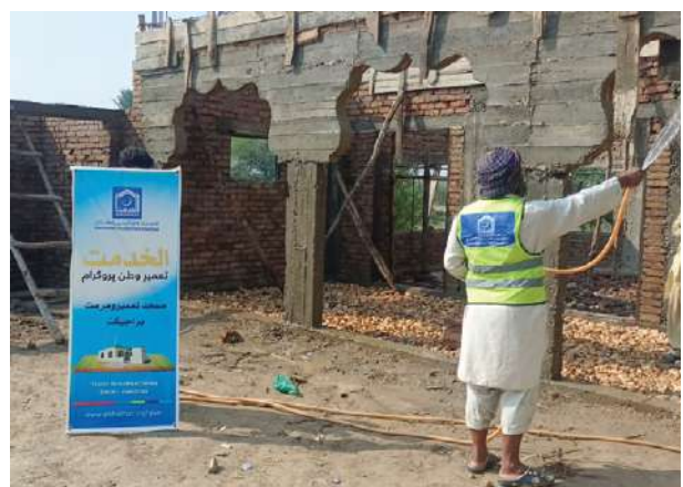
Flood-damaged Masjid is under reconstruction in Sindh.
